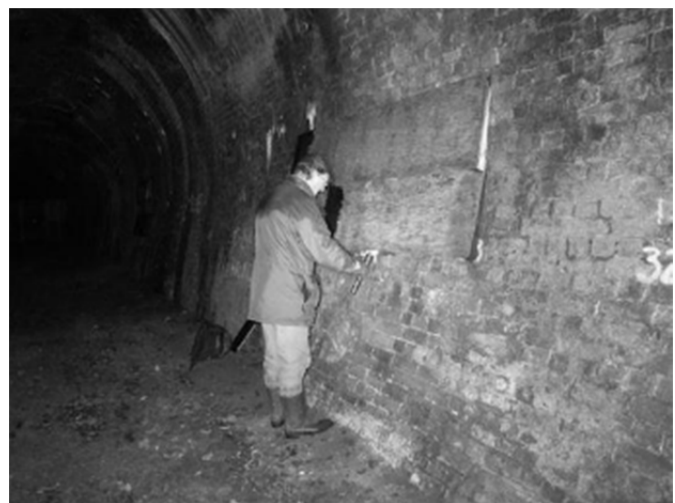
Martyn Phillis checking the boards with a mirror and torch
